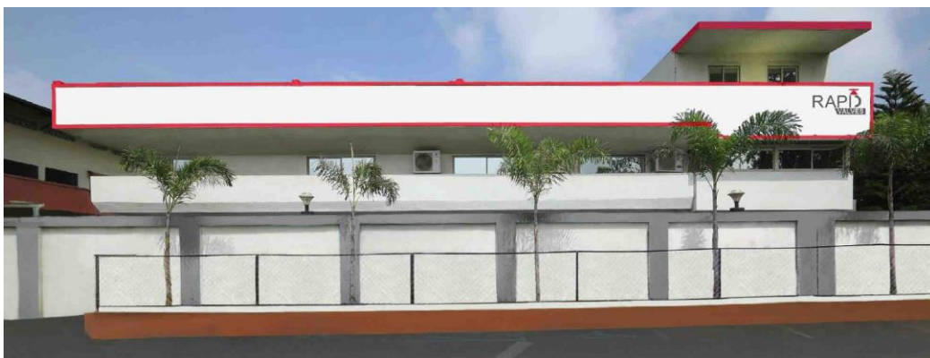
Front view of office
